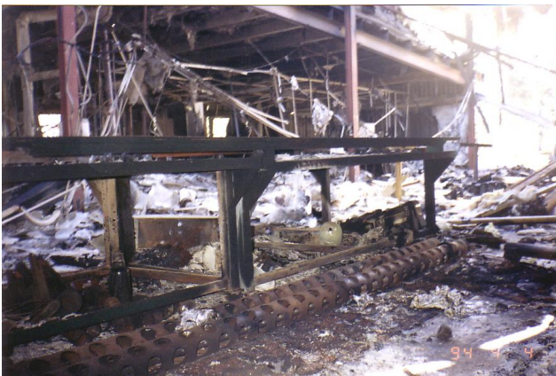
Front view of the building after explosion and subsequent fire that resulted from a barrel of methanol stored in the area, and the perforation of a gas line within the building.
