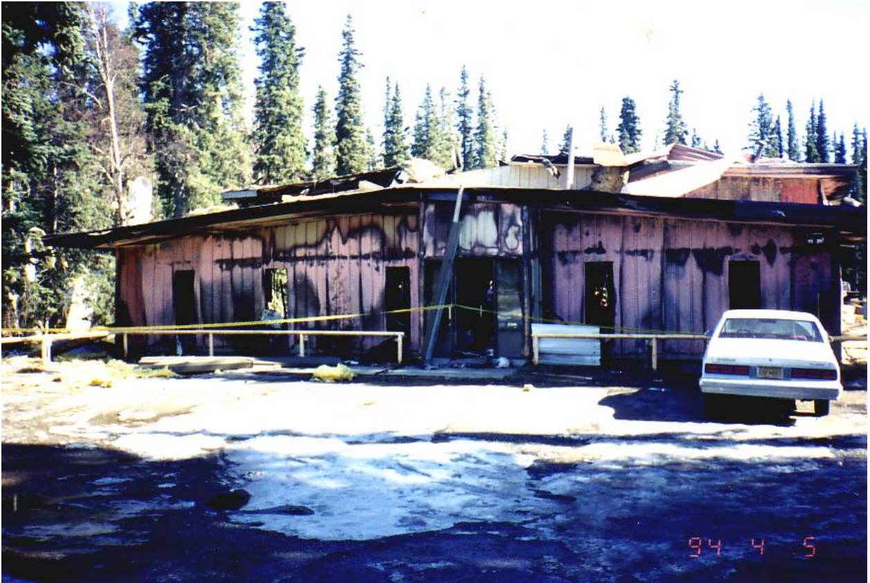
Front view of the building after explosion and subsequent fire that resulted from a barrel of methanol stored in the area, and the perforation of a gas line within the building.
