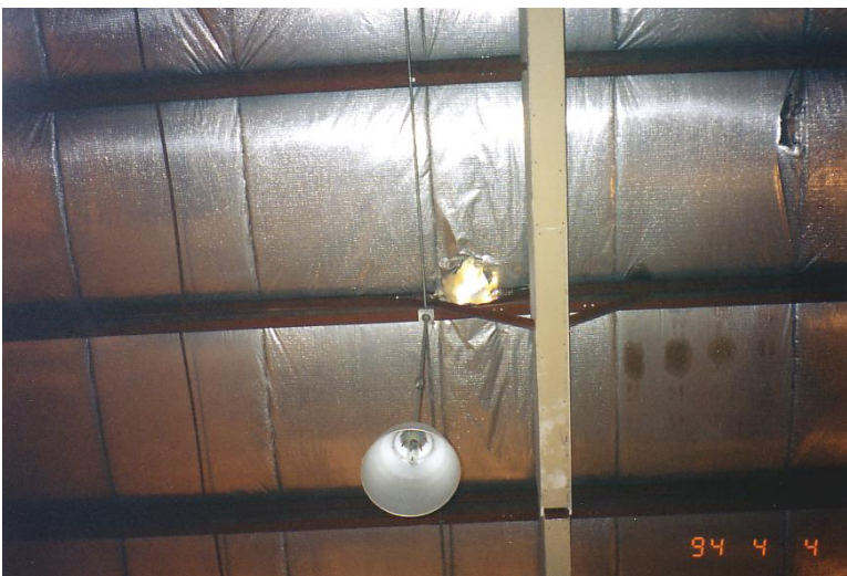
Interior view of a hole in the building's roof that was perforated by shrapnel.
