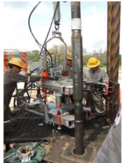
Fishbones first installation in Texas
